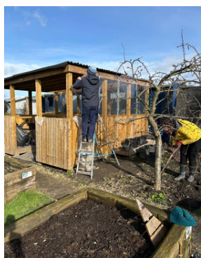
Busy at work on the plot
