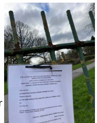
Shelter demolition notice
