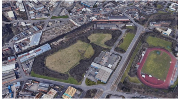
Attercliffe Waterside area
