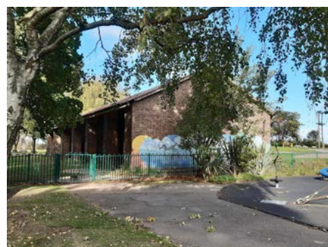
The shelter to be demolished
