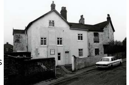
The original 'house' mosque at 13 Industry Rd
