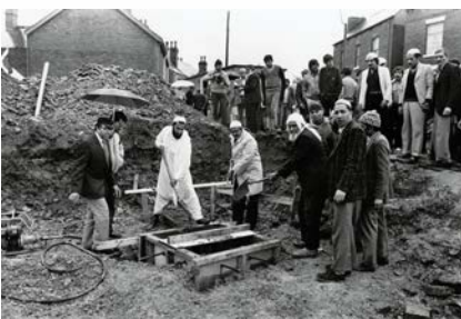
Laying new foundations of the 1984 mosque
